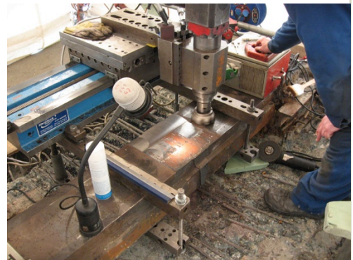
Milling of the track.
