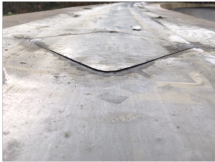
The provisional repair with the fitting piece.
