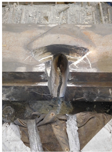
The welding is nearly completed.
